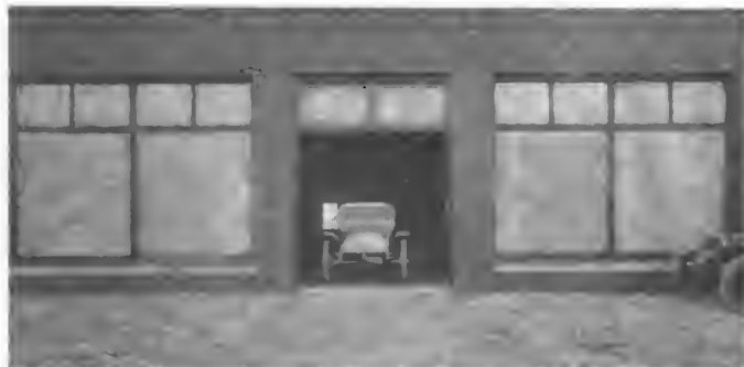
MAIN ENTRANCE BEYSTER & THORPE GARAGE, DETROIT.
